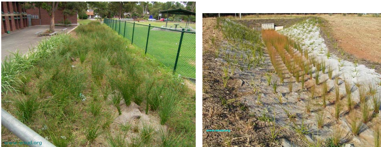
Figure 7: (Top left) Examples of Vegetated Swale (Source: Water Sensitive Urban Design of the Sydney Region)
