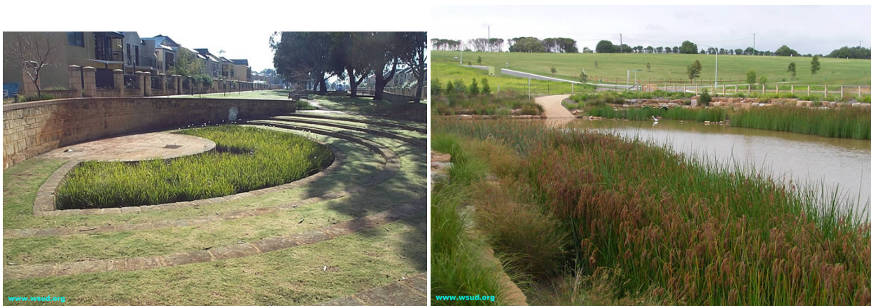
Figure 10: Example of a constructed wetland (left) and a constructed wetland within a retention basin (Source: Water Sensitive Urban Design of the Sydney Region)
