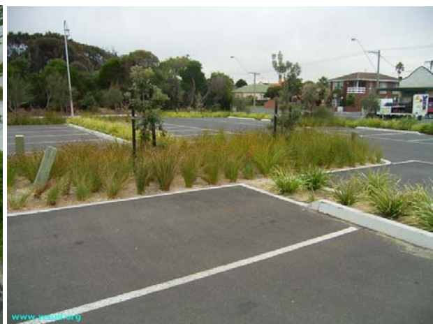
Figure 13: Infiltration trench and rain garden surrounding car parks (Source: Water Sensitive Urban Design of the Sydney Region)
