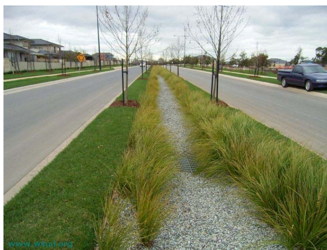
Figure 3: Example of grassed swale (top) and vegetated swale (bottom) (Source: Water Sensitive Urban Design of the Sydney Region)
