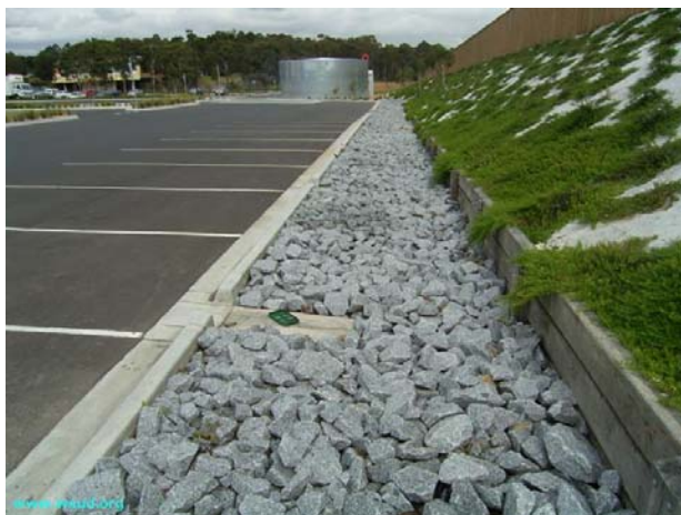
Figure 13: Infiltration trench and rain garden surrounding car parks (Source: Water Sensitive Urban Design of the Sydney Region)
