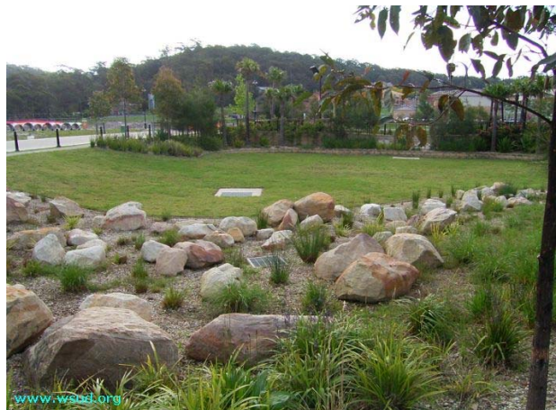
Figure 9: Examples of Bio-Retention Basins (Source: Water Sensitive Urban Design of the Sydney Region)
