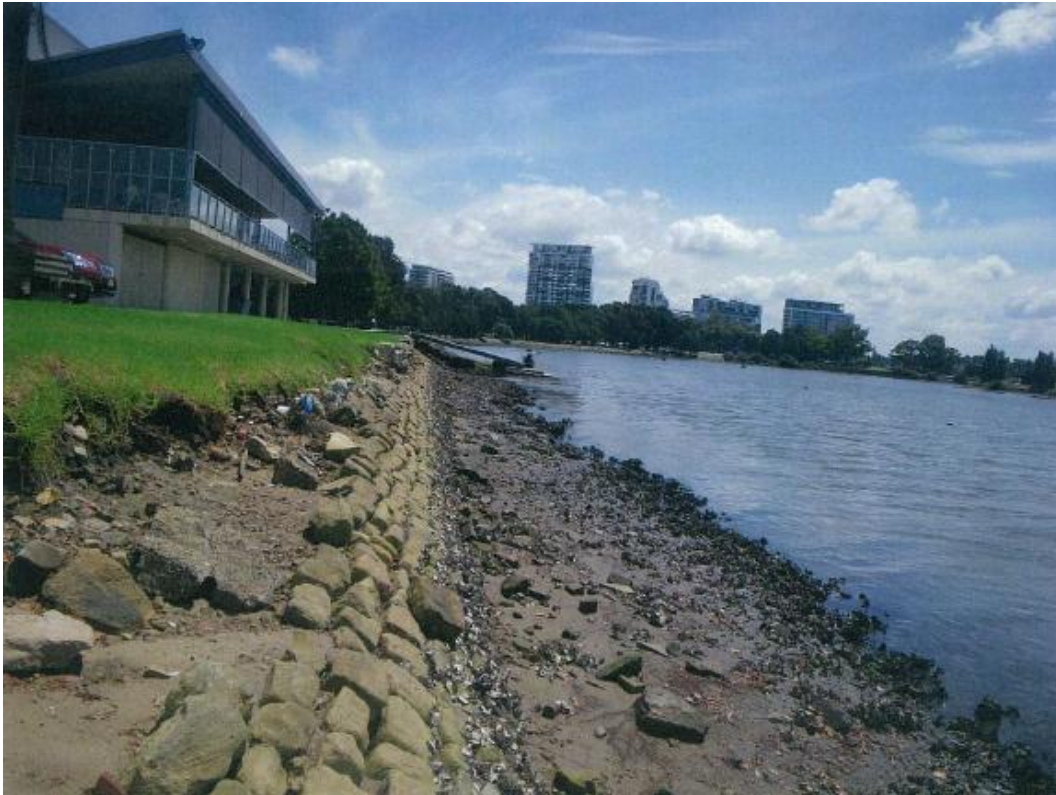
Figure 13 Example of deteriorated channel on the Cooks River (Source: Rockdale Council)
