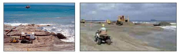
Figure 6.2 Nourishment Campaign Using Pipeline Delivery Method
