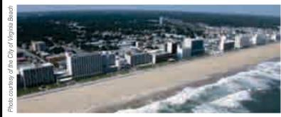
An estimated \$105 million in damage was prevented after Hurricane Isabel struck a nourished beach with a seawall at Virginia Beach in fall 2003.<sup>7</sup> The project was designed to stop a 9-foot storm surge – and it did. The nourished beach minimized wave attack and overtopping of the seawall, the community's last line of defense.
