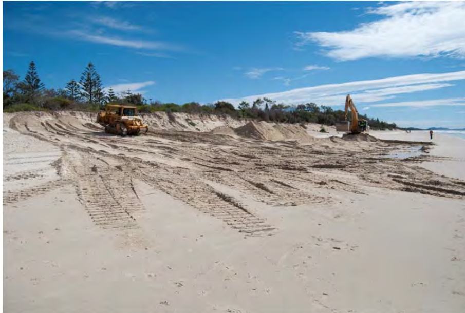
Fig. 3. Beach scraping works showing its extent and impact on New Brighton beach (Photo: S. Smith).
