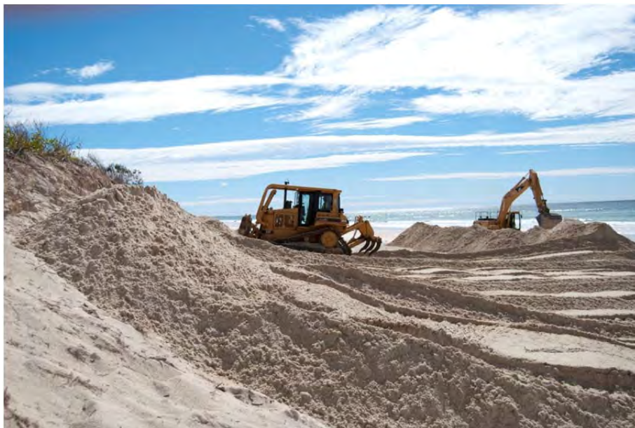
Fig. 2. Sand was pushed to the top of the beach to widen the dune (Photo: S. Smith).
