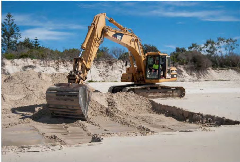
Fig. 1. A backhoe removed the top 0.2-0.5 m of sand from the beach at New Brighton (Photo: S. Smith).
