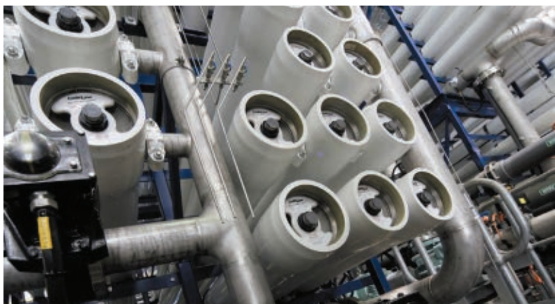
An example of reverse osmosis membrane technology used for the desalination of seawater.
