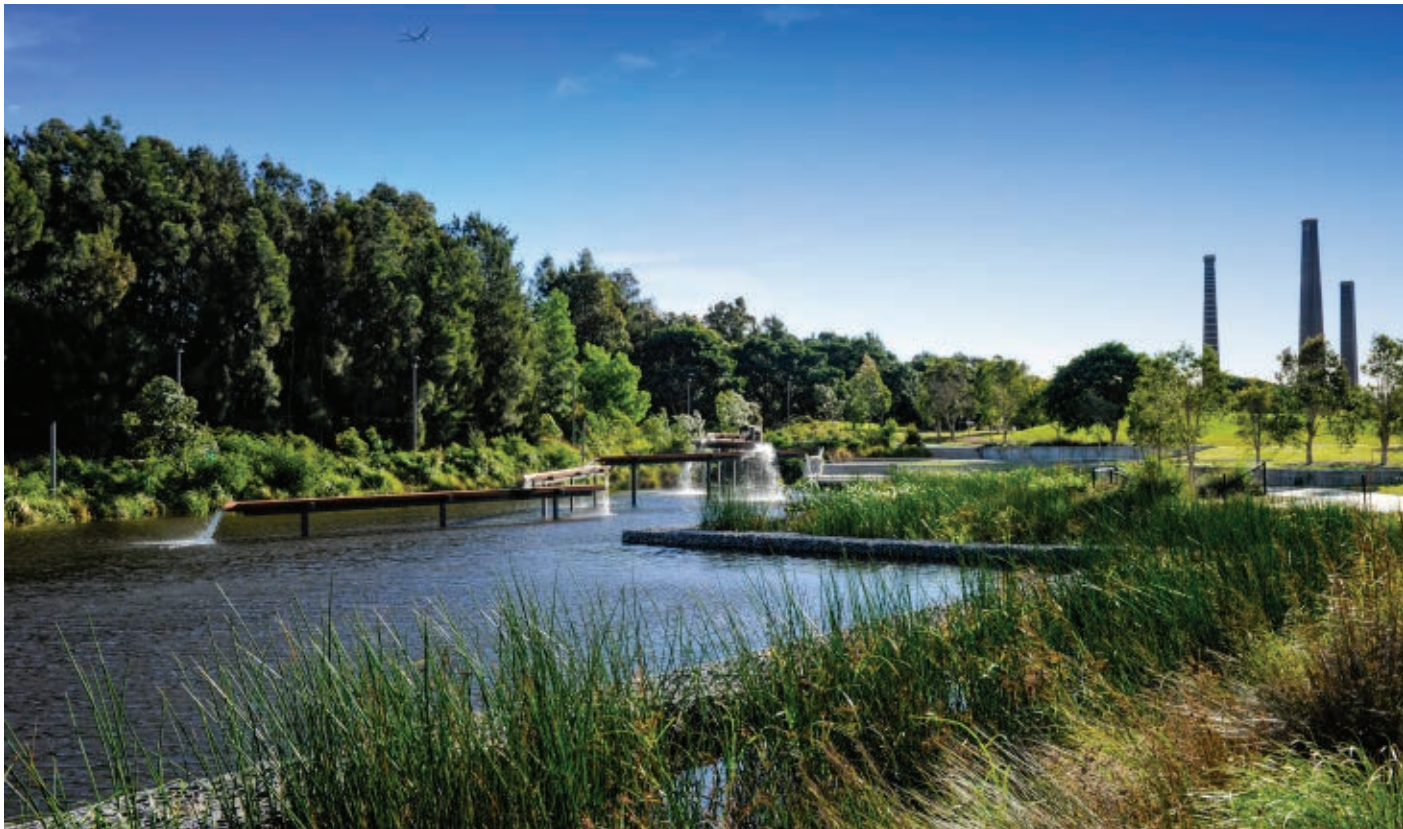
Sydney Park stormwater harvesting, providing unrestricted irrigation of playing fields, passive recreation areas and forested areas in a high-density inner city area.
