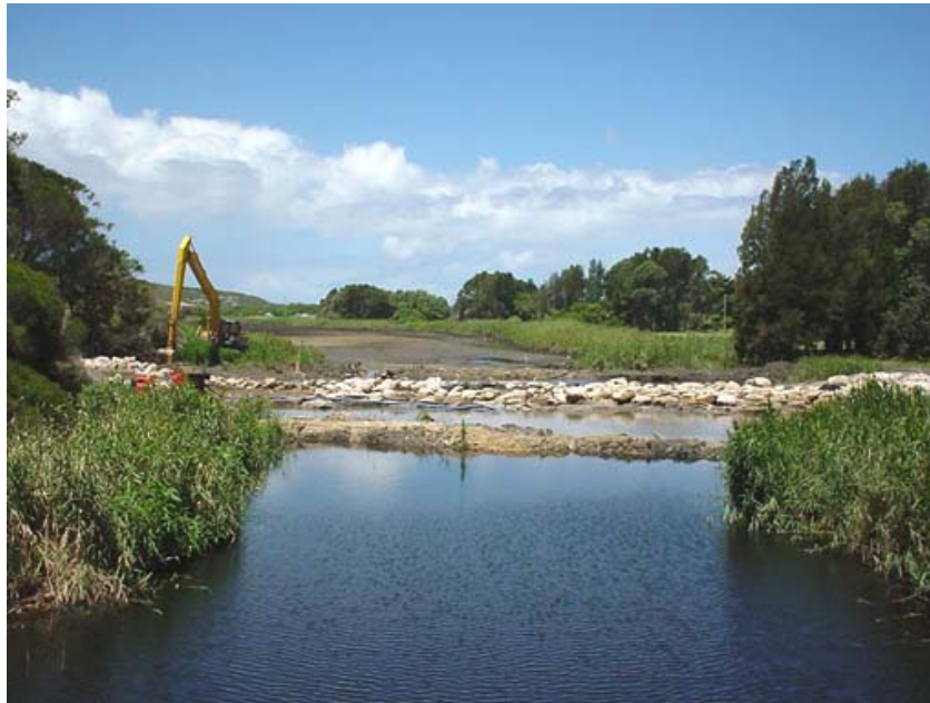
Wetland restoration works, Curl Curl Lagoon, Warringah Shire
