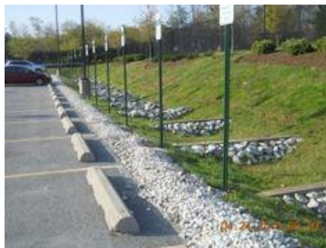
Figure 28: Grass swale with check dams
