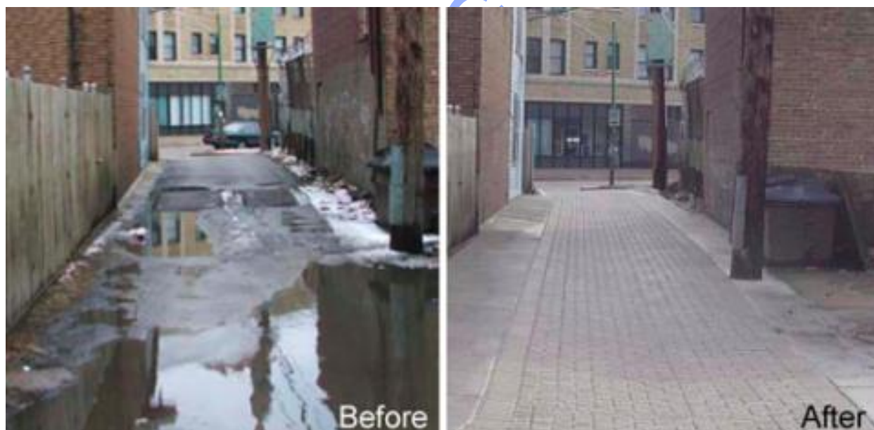
Figure 24: Before and after images of an alley in Chicago which showed chronic signs of flooding until replaced by permeable pavers and surfaces that allow water infiltration (Economides, 2014).
