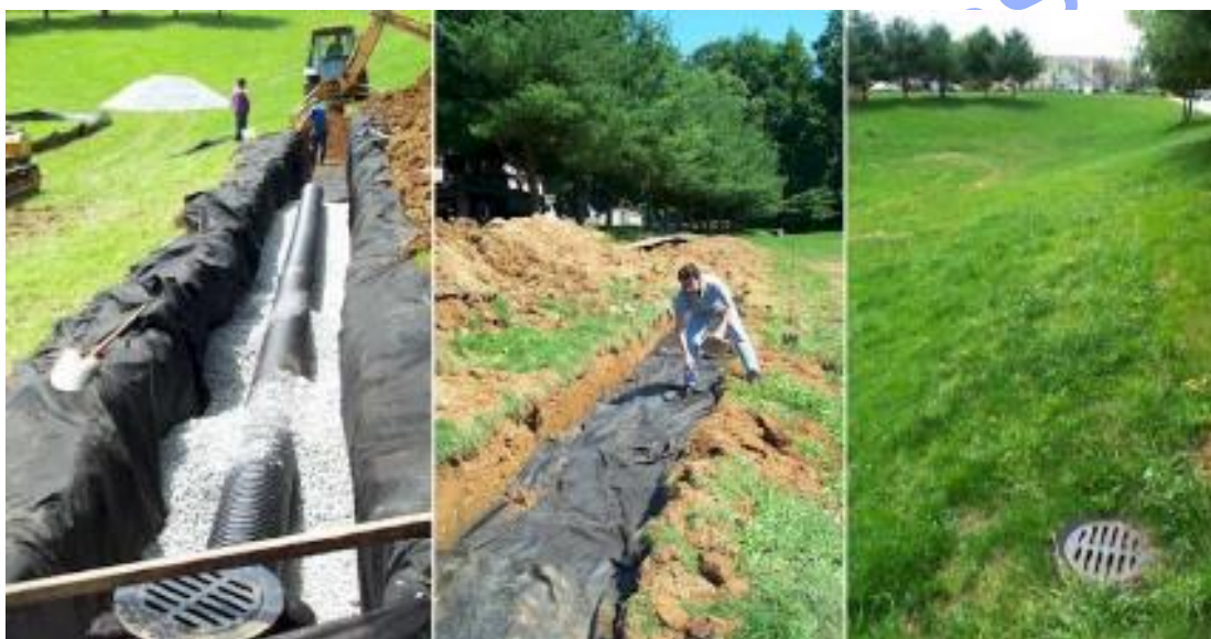
Figure 30: Infiltration trench (Pennsylvania Department of Environmental Protection, 2006)
