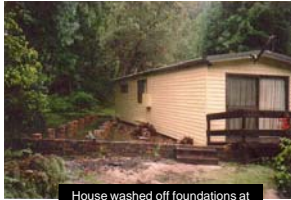
House washed off foundations at Great Mackerel Beach 1989
