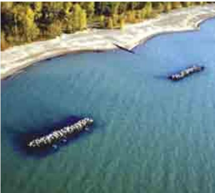
■ Breakwaters, constructed offshore but parallel to the shore, break waves before they reach the shore. Breakwaters help retain sand and reduce local erosion.
