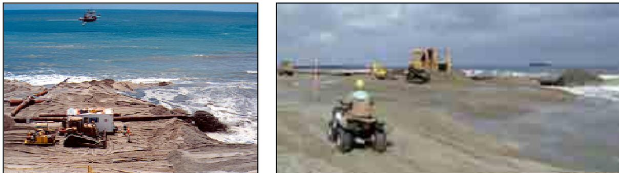
Figure 6.2 Nourishment Campaign Using Pipeline Delivery Method
