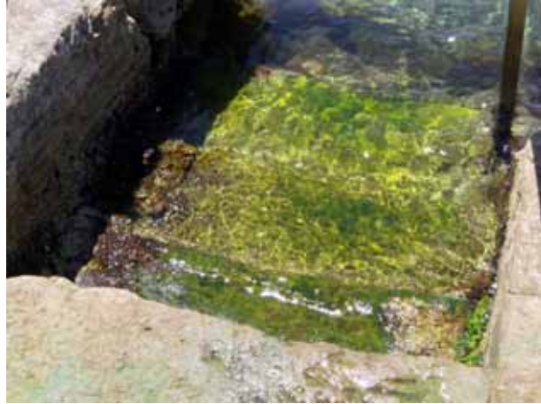
Photo 7 – Steps in Mahon pool heavily fouled by green algae
