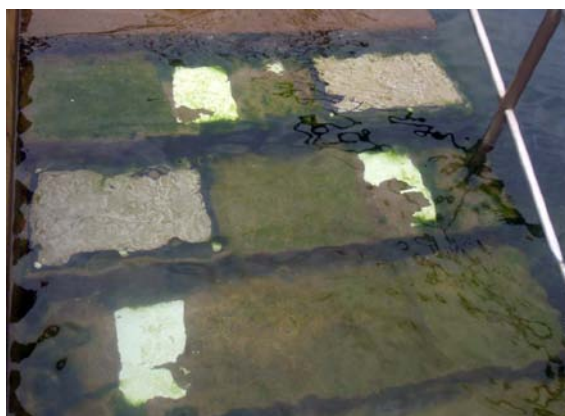
Photo 10 – Steps at 6 weeks. Algae have grown back on concrete areas cleaned 2 weeks earlier by jet-blaster and there is less algal growth on SW mats and white-X8 coating than at 4 weeks (see Photo 9). Recent 'big seas' appear to have 'self-cleaned' SW mats and white- X8 coating on steps (compare with Photo 9B).
