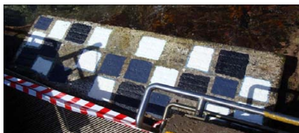
Photo 1 – Clovelly Step at 0 weeks. The direct application of 4 coatings (white-X8, black-Y3 and blue-Z3, white-X7 squares [flaked off in first week]) onto concrete step. The control squares are untreated concrete.
