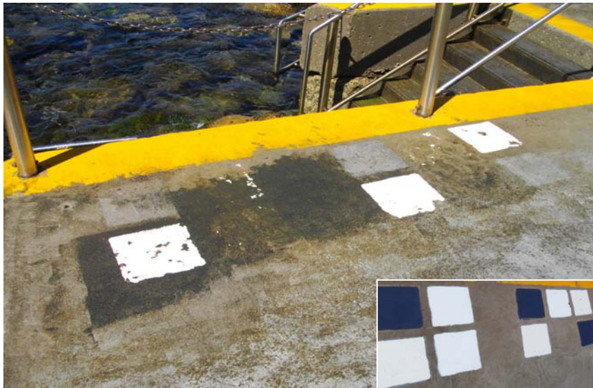
Figure A.2 Test area on the Clovelly promenade after 12 weeks. The surrounding area was cleaned 3 times with a high pressure water jet during the trial period. Inset: Test area at the start of the Trial.
