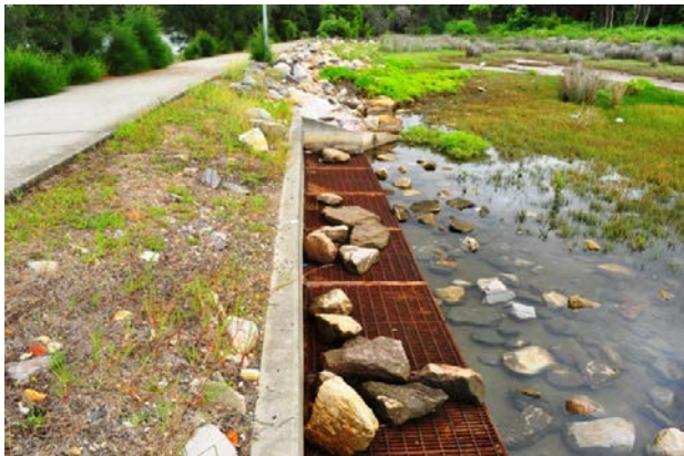
Figure 58. Tempe Saltmarsh, Cooks River. Under/Over Inlet Structure
