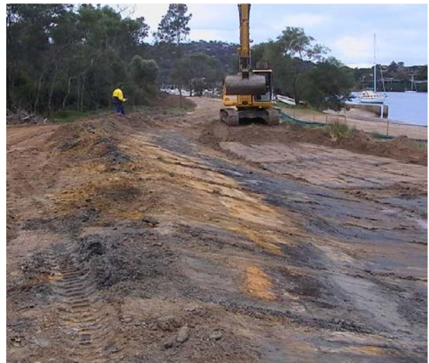
Figure 61. Kooroowall Reserve Creating saltmarsh inundation area.
