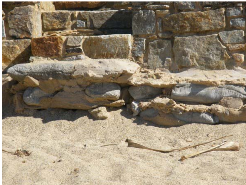
Figure 6 Private seawalls can be constructed as a landscape feature without due consideration to storm loadings. This elevated toe is exposed above the HWM on the public beach
