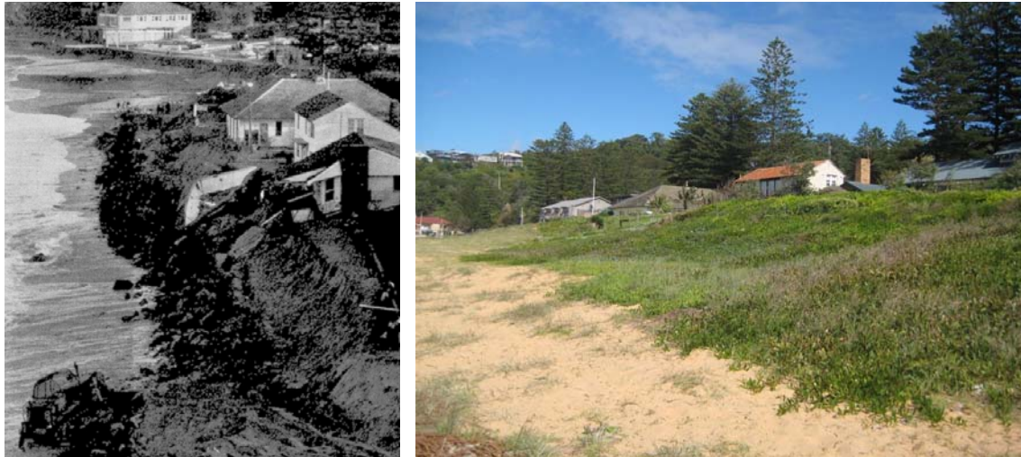
Figure 3 A substantial rock armoured seawall has been constructed following storm erosion and is now buried beneath this revegetated sand dune
