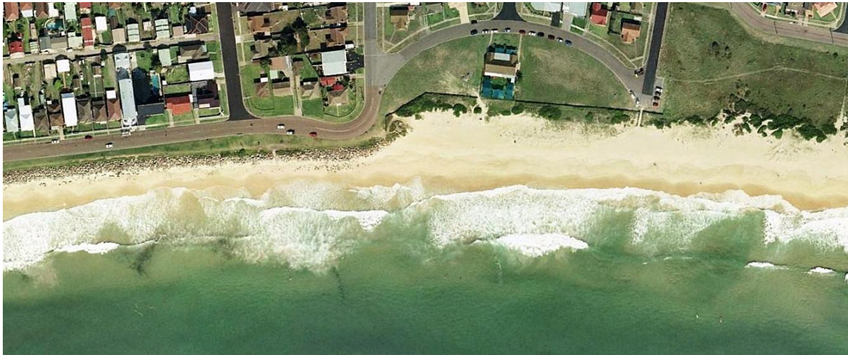
Figure 7 Increased erosion commonly results adjacent to the ends of a seawall (end effects) as a result of the sand deficit moving alongshore past the seawall and the loss of sand supply from the now protected dune
