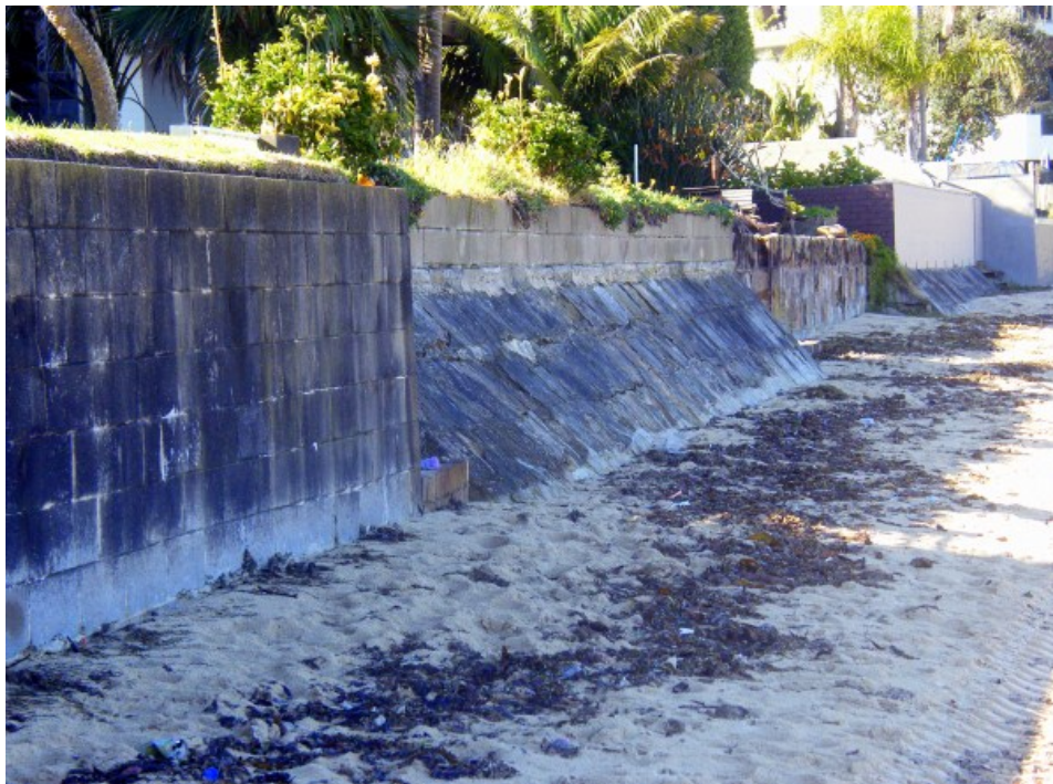
Figure 4 A variety of private seawalls constructed to varying designs and standards along private property boundaries in Sydney Harbour
