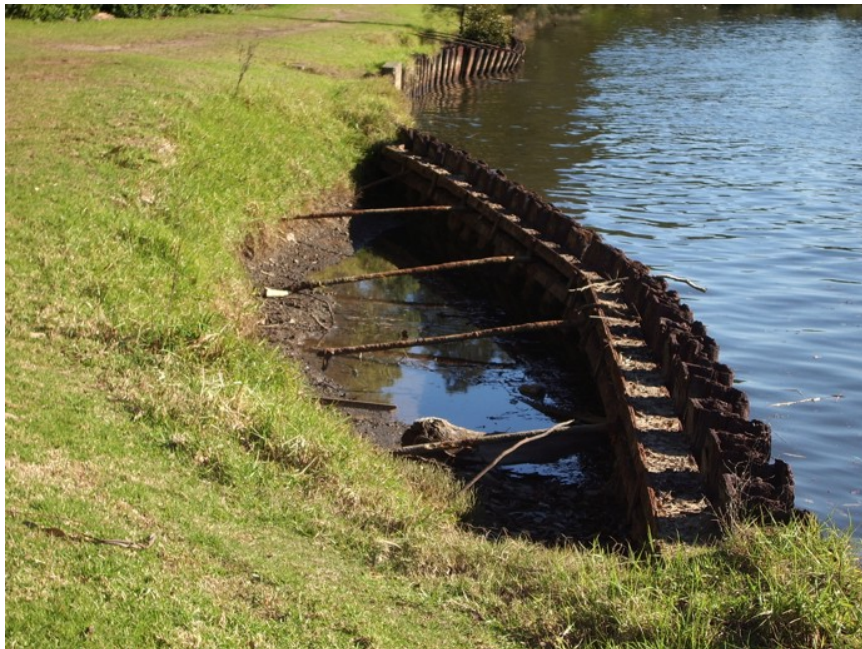
Figure 2 Often the failure or partial failure of a seawall or revetment is obvious. At other locations they may not even be visible except during storm events
