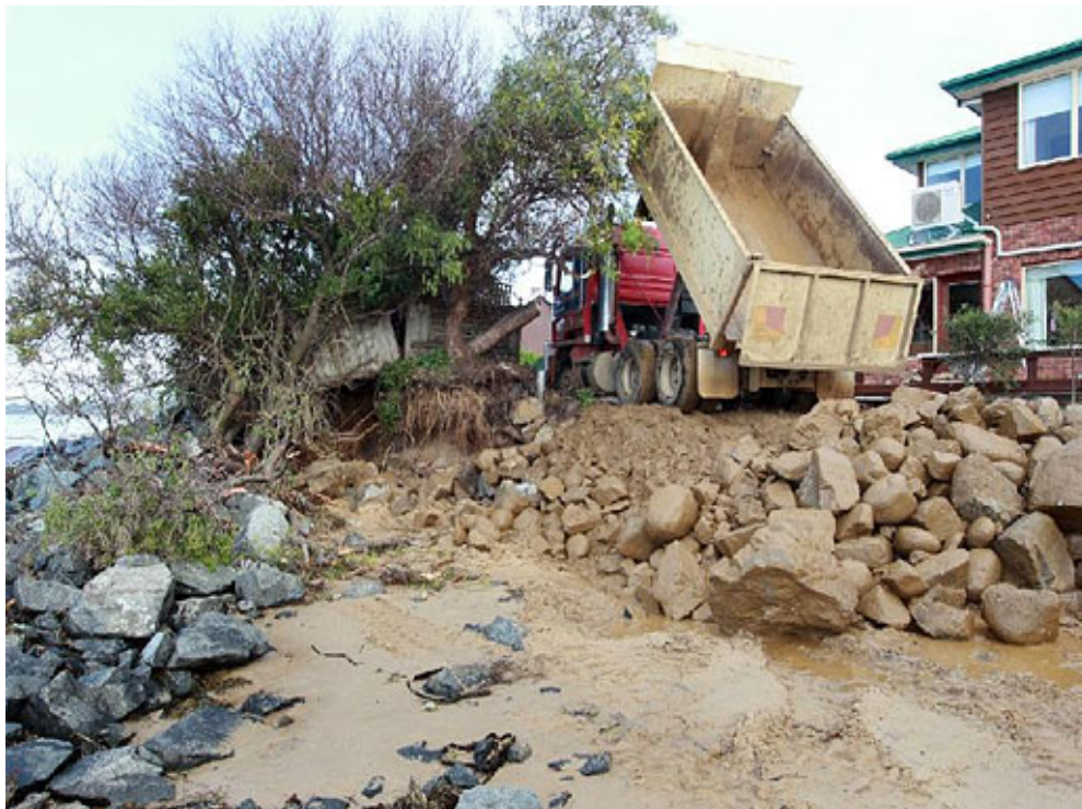
Figure 5 Many seawalls are constructed during storms as an emergency response to the threat posed to existing development. Few are ever removed once the threat has passed
