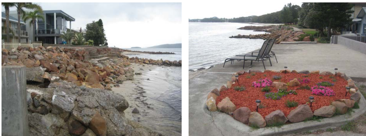
Figure 11 Ad hoc coastal protection works and landscaping constructed seaward of the property boundaries with resulting loss of the once sandy beach and public foreshore access
