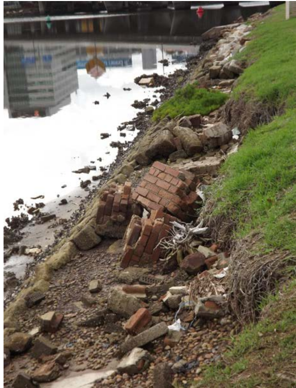
Figure 12 The historic existence of a seawall or revetment should not necessarily result in the structure being upgraded or even retained
