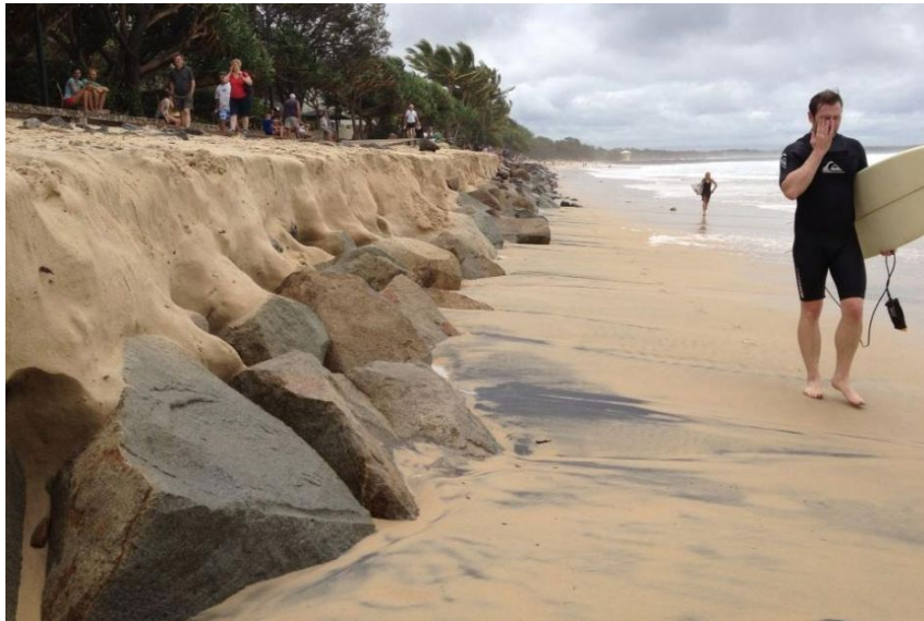
Figure 10 Erosion exposes the crest of a buried seawall which was not visible prior to the storm. The structure and level of the toe are not readily discernible
