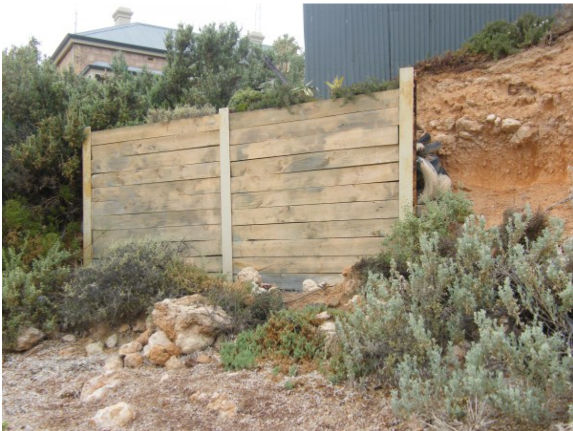
Figure 9 A steel pile and timber plank, cantilevered seawall constructed at the back of the public beach. Erosion behind the wall is backfilled with car tyres
