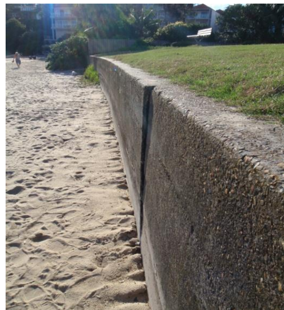
Figure 3 Toe bearing failure schema and illustration showing incipient failure
