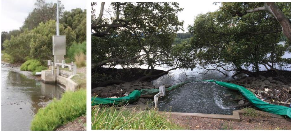
Figure 5.1: Slip gate (left) and boom (right) at Badu Wetland (Bowie, 2015)
