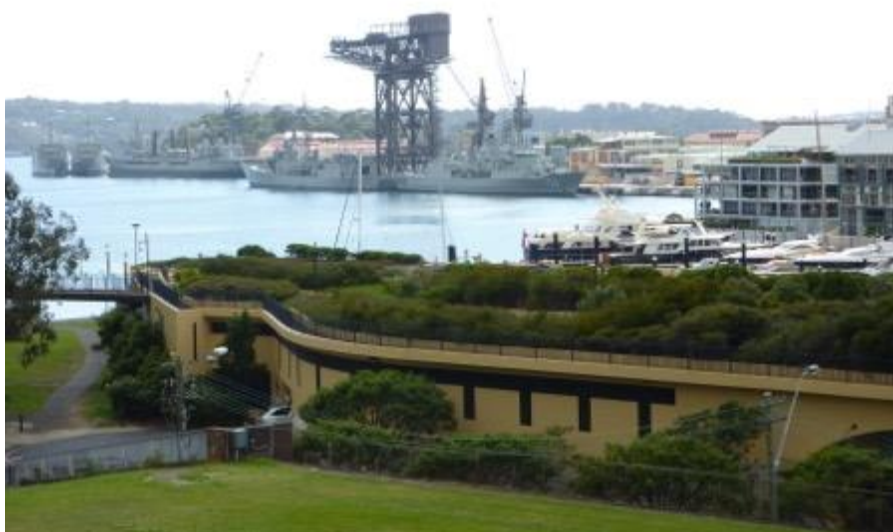
Green roof vegetated with a mix of mainly native shrubs provides habitat on an apartment complex in Woolloomooloo
