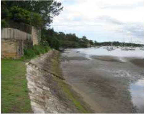
Inner harbour sea walls
