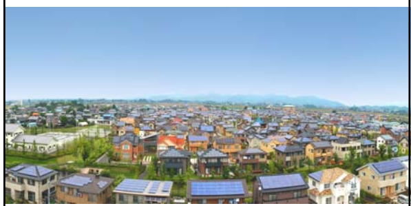
Ota, Gunma, Japan - over 500 houses totalling 2,16 MWP
