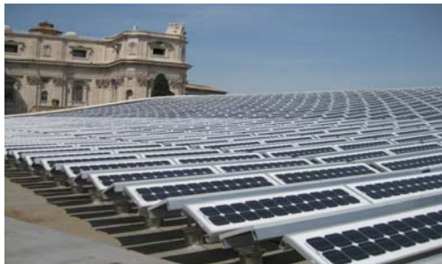
221kWp of blessed Vatican PV
