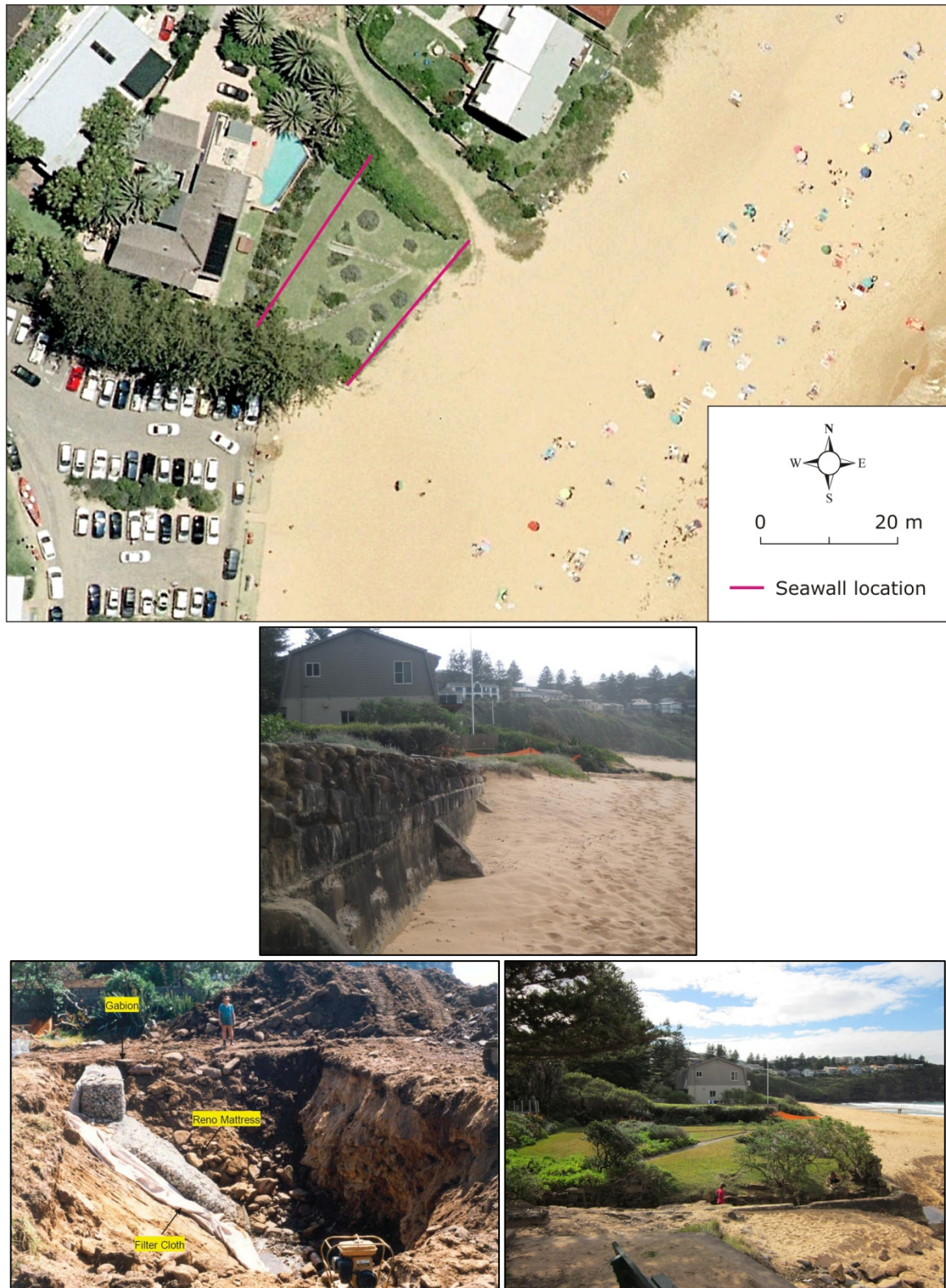
Figure 2.4 Bilgola Beach Seawalls 2A and 2B Fronting 21 Bilgola Avenue
