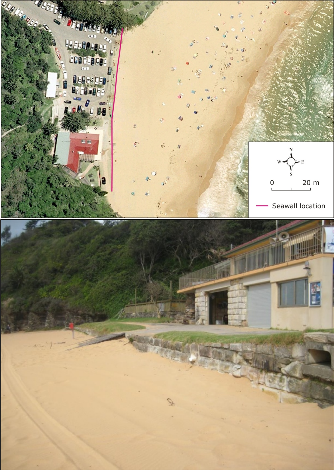
Figure 2.5 Bilgola Beach Seawall 3 Fronting Bilgola SLSC 10 April, 2012
