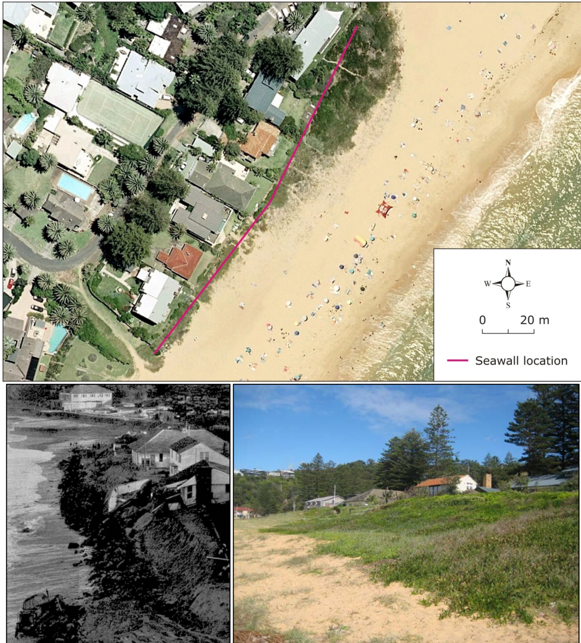
Figure 2.3 Bilgola Beach Seawall 1 Fronting Allen Avenue Properties
