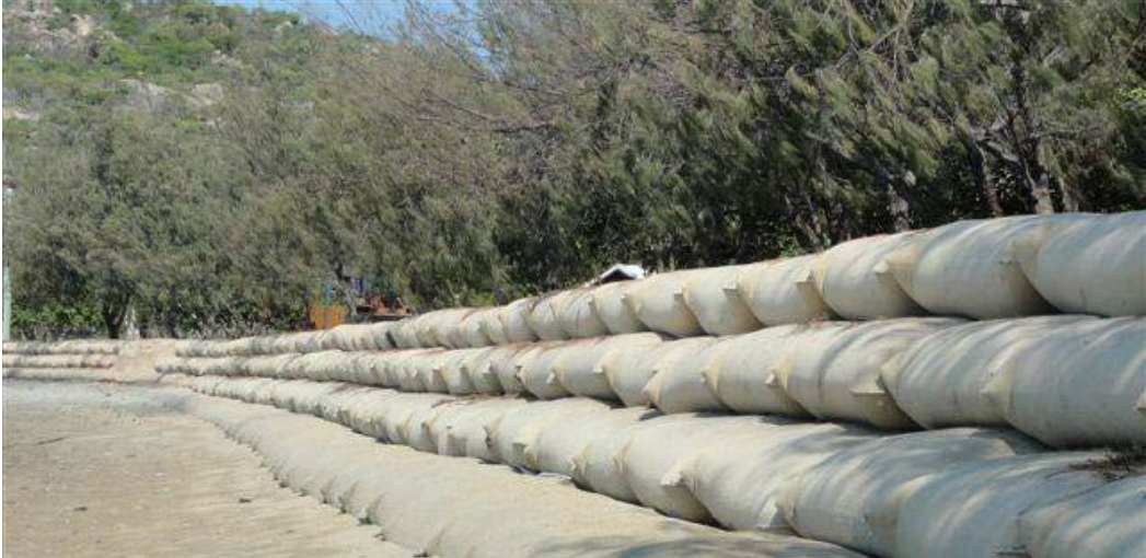
Figure 9 Sandbag gravity seawall (source: Geofabrics Australasia)
