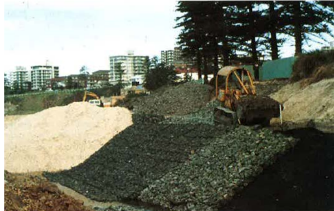
Figure 13 Sloping Reno-mattress dune revetment under construction
