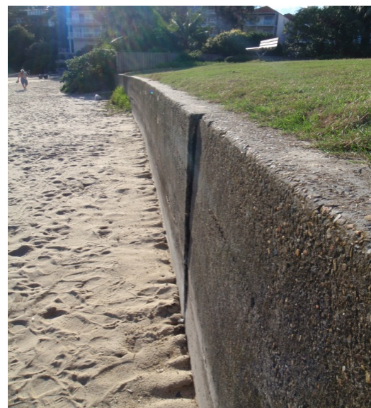
Figure 19 Toe bearing failure schema and plate showing incipient failure
