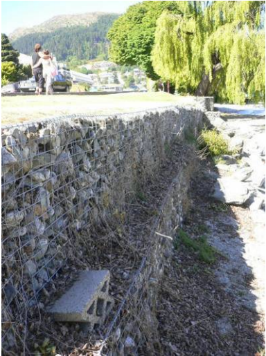
Figure 10 Flexible near-vertical mass gravity seawall Left: Rock boulder gravity seawall; Right: Gabion gravity seawall (Source: Deborah Lam)
