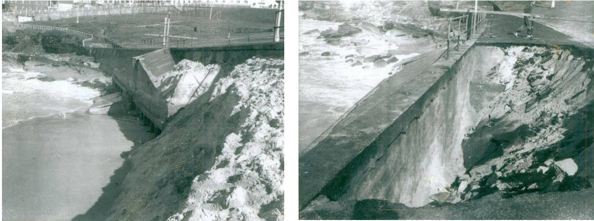
Figure 18 Loss of backfill of mass gravity seawall at South Bondi Beach 13 June 1974 as a result of toe scour and undermining of the footing
