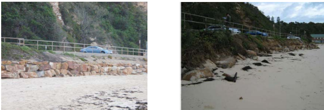
Figure 21 Blockwork gravity wall failure
