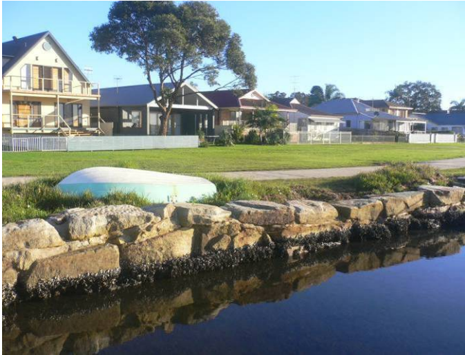
Figure 10 Flexible near-vertical mass gravity seawall Left: Rock boulder gravity seawall; Right: Gabion gravity seawall (Source: Deborah Lam)
