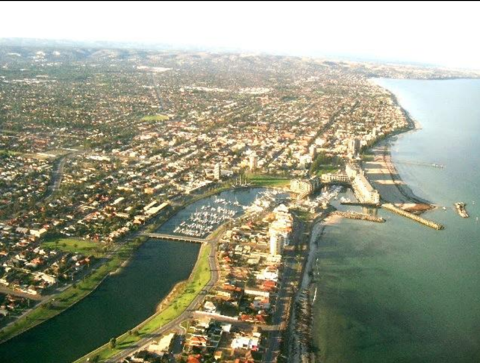
Glennelg bypass with dredging and pumping
