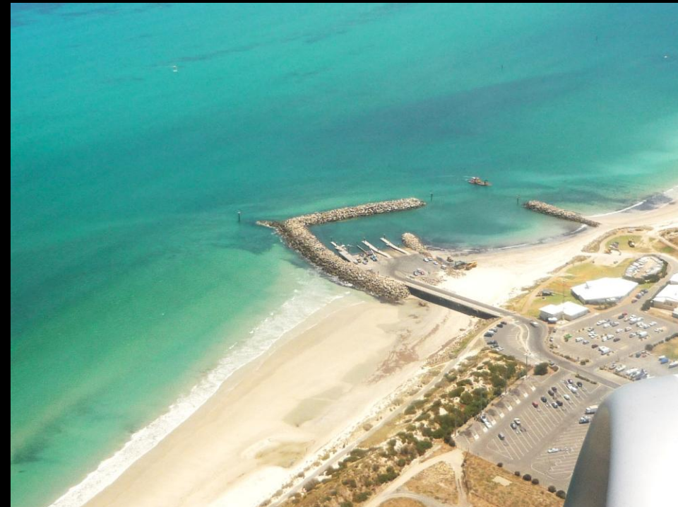
West Beach bypass with dredging and pumping
